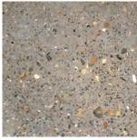
Polished concrete floor slab with exposed aggregate finish
