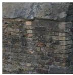
Example of Gault brickwork used for previous Guildhall buttress repairs
