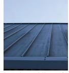
Zinc standing seam cladding to roof dormers
